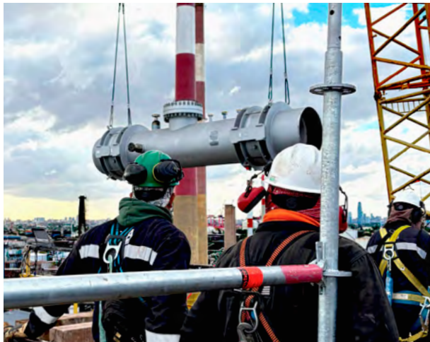
FCC Expansion Joints Installation Supervision in Argentina
