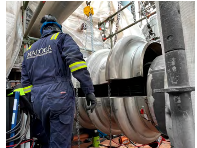
High-Pressure Clamshell Expansion Joint in Alloy 625 for Petrochemical Plant in Europe
