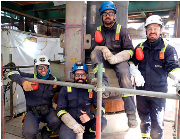
FCC On-Site Service at UK Refinery.
