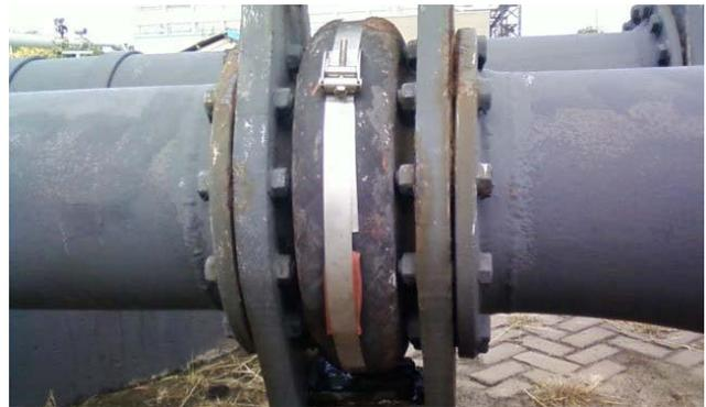
Expansion joints rating for temperature, pressure, vacuum and movements must match the system requirements. If the system conditions exceed those of the expansion joint selected it may be a cause of failure. It is important to review the piping system layout, medium, pressure, temperature, movements, and other items which may affect the performance of the expansion joint.
