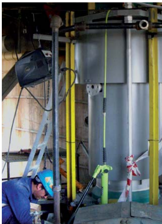
On-Site Inspection at BPOil Refinery
